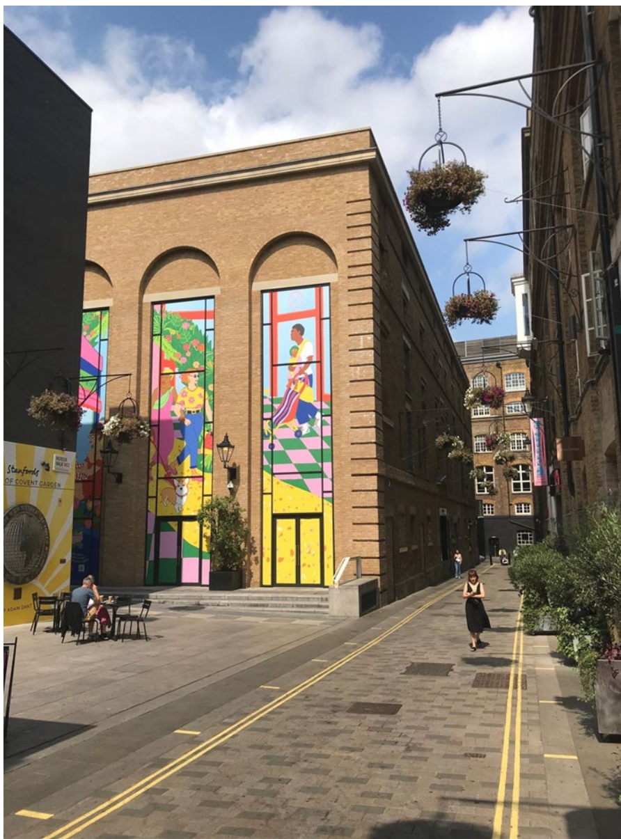
1 Mercer Walk, Langley Street
